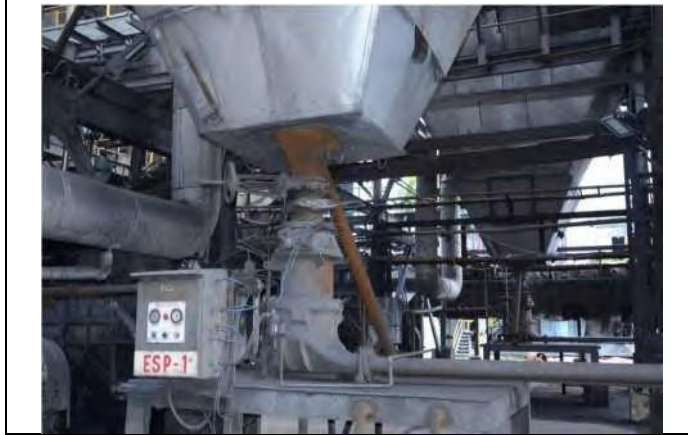
Dense phase pneumatic ash handling system
