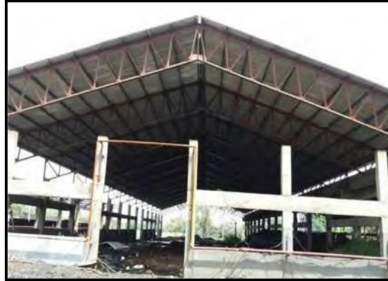
Shed for coal storage
