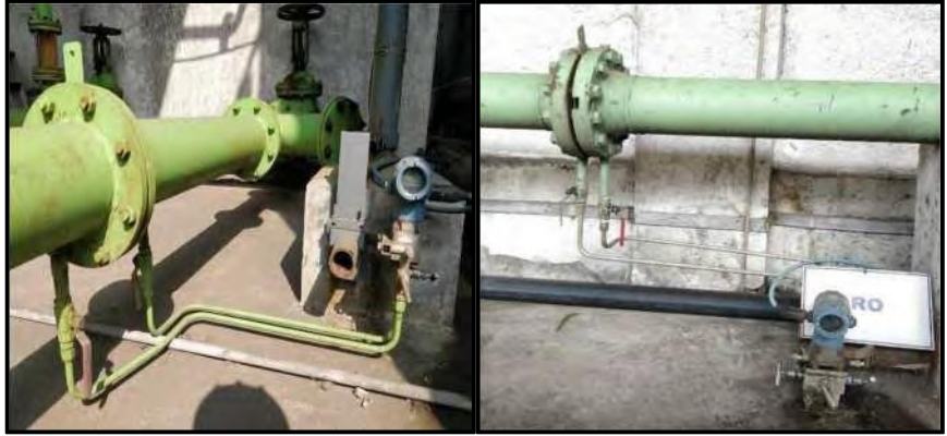
Water meter @ Inlet line
