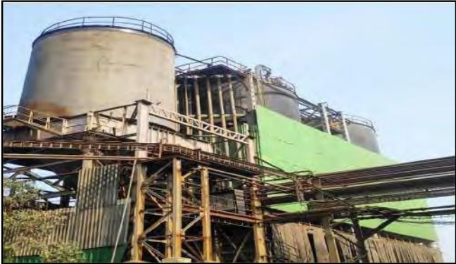
Photograph of Closed silos for Fly ash / Bottom ash storage:-
