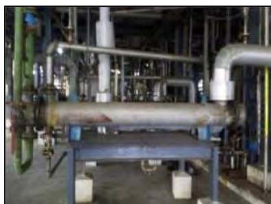
a) Condensers at Solvent Recovery
